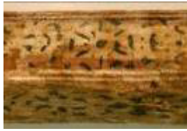
Lübeck, Depenau 35, Deckenbalken, 1612-14
